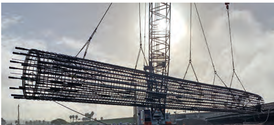
Heavily instrumented rebar cages in San Diego
