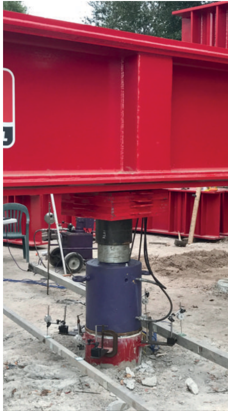
The Georgia test involved jack loads from two 40 in (102 cm) beams
