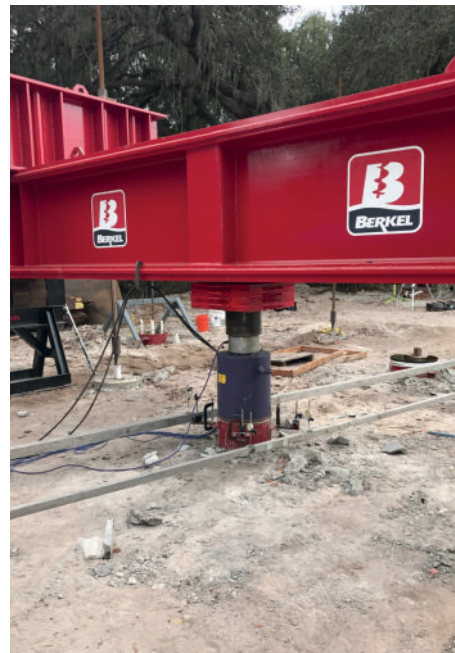
High capacity D1143 load test in Georgia
