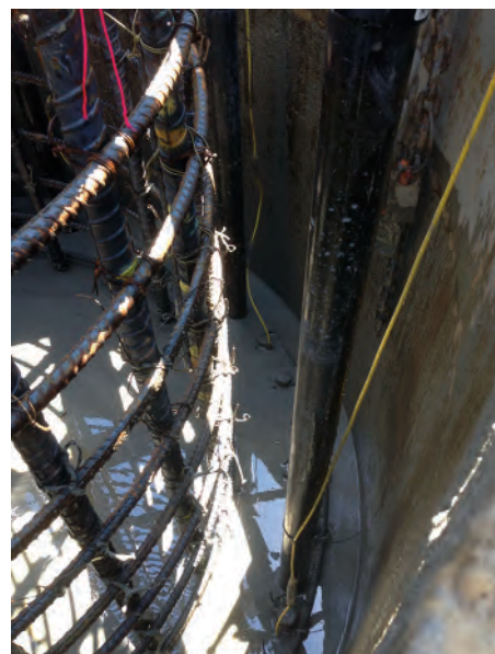
Shaft instrumented with TIP wires for a SCDOT project
