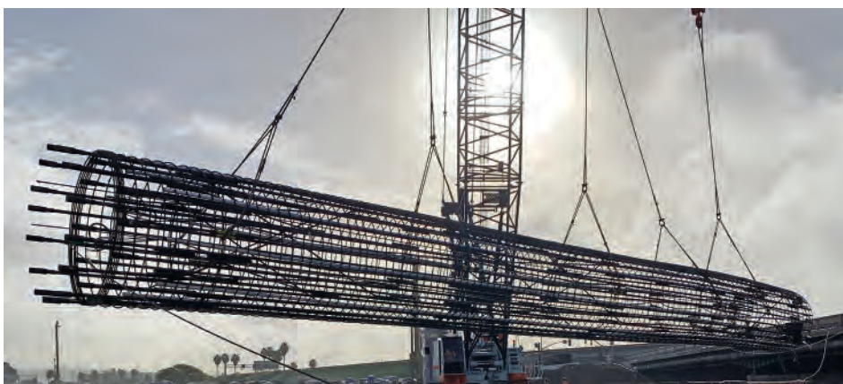
Heavily instrumented rebar cages in San Diego
