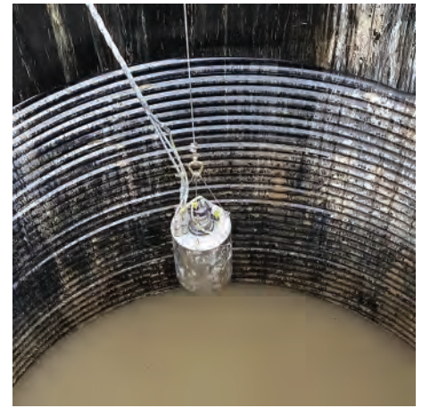
Shaft inspection devices (SIDs) can aid engineers as they try to verify tip conditions.
