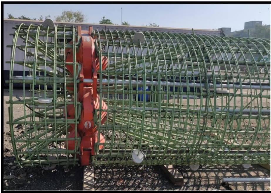
Figure 3 – (Sakhuja et. al. 2019 Figure 8 – Positioning of Jacks in the Pile Cage)
