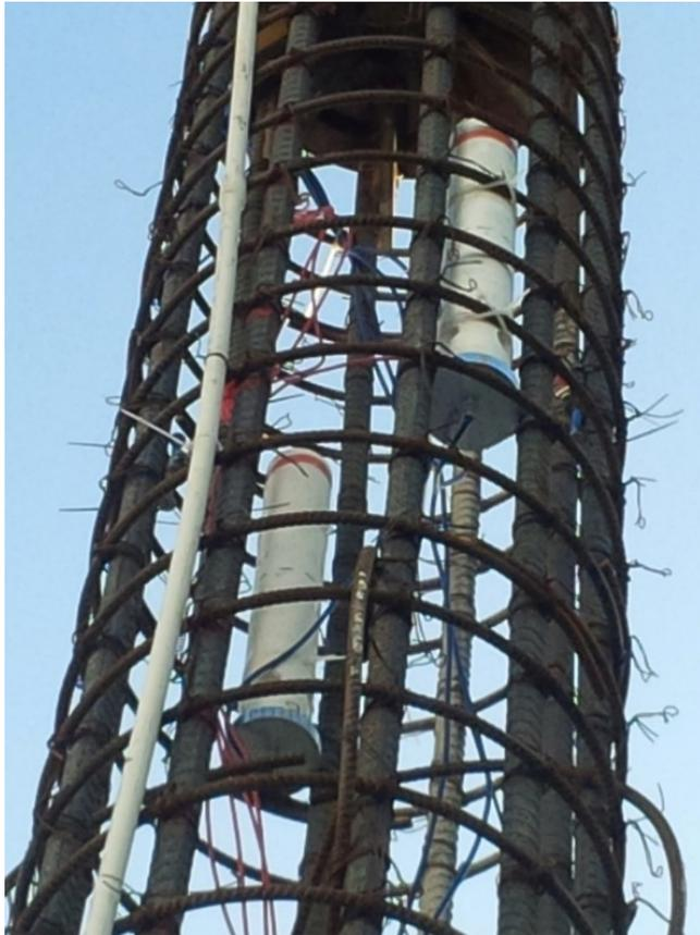
Figure 6. CSM pair in rebar cage below jack – Project B
