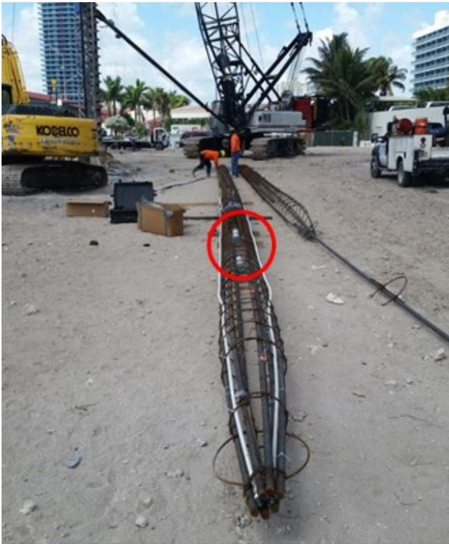
Figure 4. CSM pair in rebar cage (circled) – Project A
