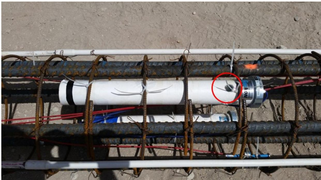
Figure 3. Self-filling (“a”, top) and pre-filled (“b”, bottom) CSM mounted in rebar cage (vent holes in self-filling tube circled) – Project A
